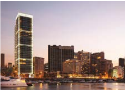
Platinum Tower, Beirut, Lebanon
